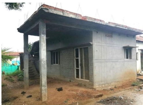
Figure A 6.3: Asha and Kumaraswamy’s House under Construction – Indira Awas Yojana
